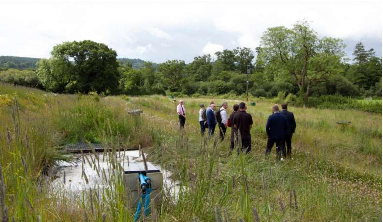
Figure 6. Constructed wetland and the 'beehive' structures which house the aeration pumps that are said to increase the removal rate of COD and organic contaminants, allowing for a faster turnover.
